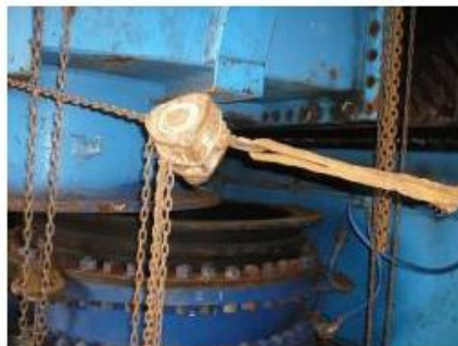
(6)查漏後水箱端蓋回裝
