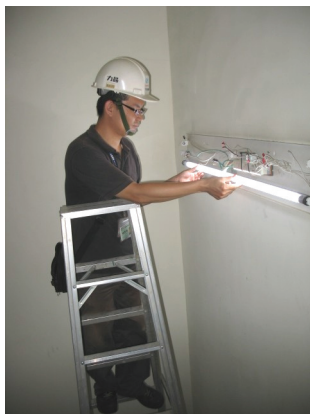
LED 燈管 DIY 安裝
