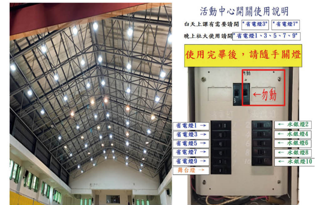
老舊燈具汰換成 LED 燈
