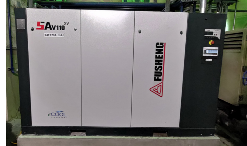
儀表及廠用空壓機更新
