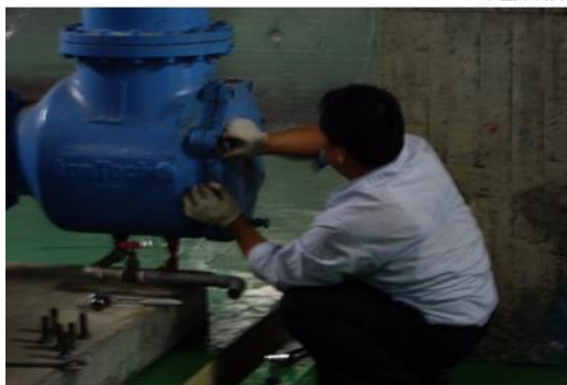
(1)拆卸過濾網蓋板
