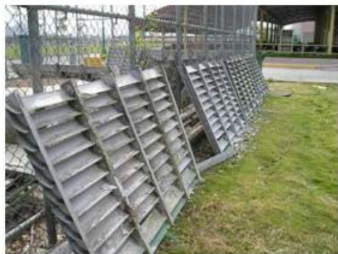
拆下冷卻水塔導流板清除水垢
